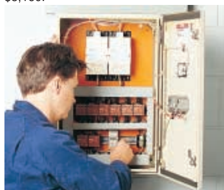
2 C-Bus four channel relays were used to switch lighting at required thresholds
