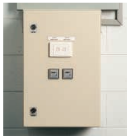
Master C-Bus switch provides total control of all factory lighting from one location
