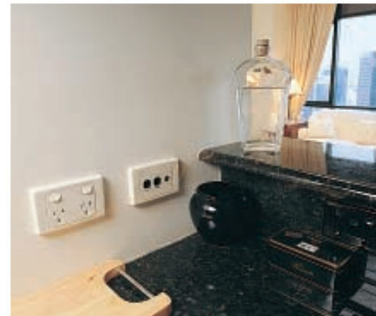
Functions can be reprogrammed at the computer interface point, situated above the kitchen bench.
