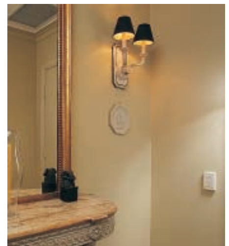
"Welcome Home" Scenario activates lights, floor heating, towel rail and airconditioning.
