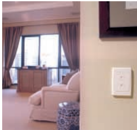
Each C-Bus keypad can dim lighting up or down when pressed for 1.5 seconds.
